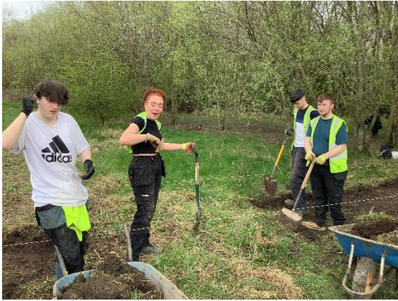
Digging the wildlife pond
